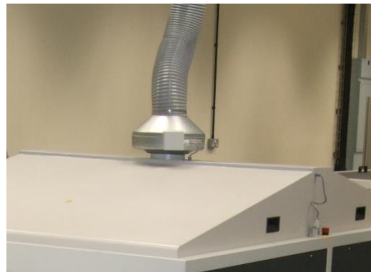
Exhaust fan extracts fumes and excess heat to provide an optimum working environment
