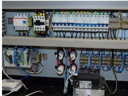
PLC control system with inverter conveyor/drive motor control
